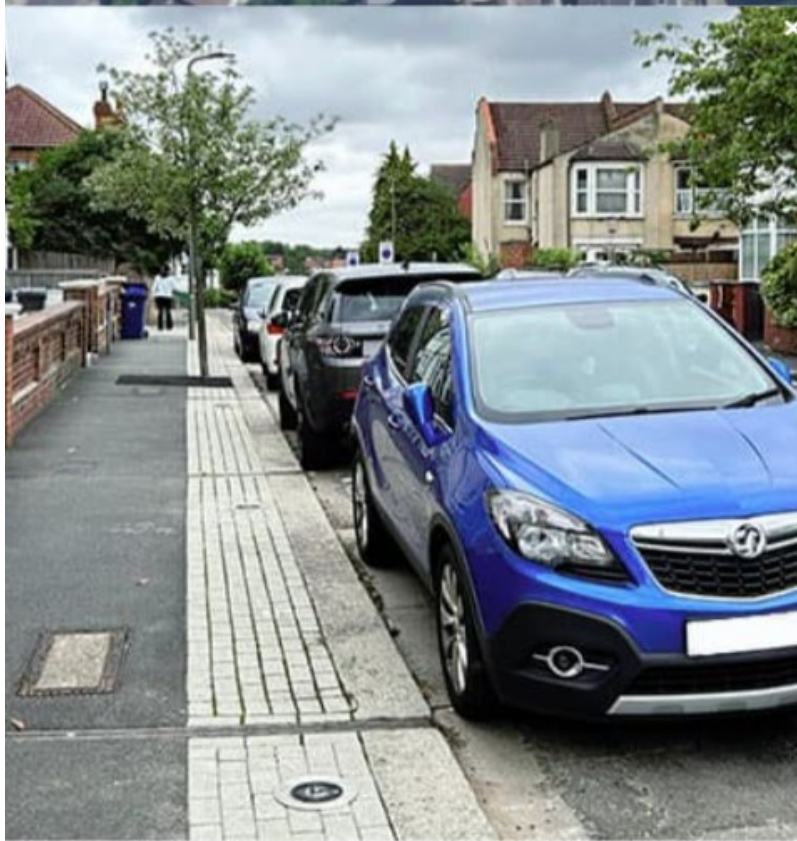
Montagu Road 1 7 Trojan charge points
